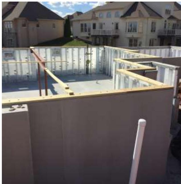
Figure 4: High Performance Homes Precast Concrete Foundation
