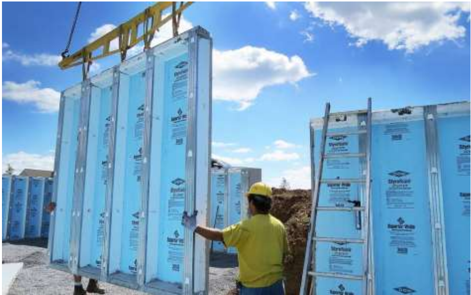
Figure 1: Superior Wall Engineered Precast Concrete Wall
