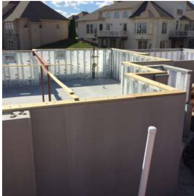
Figure 4: High Performance Homes Precast Concrete Foundation
