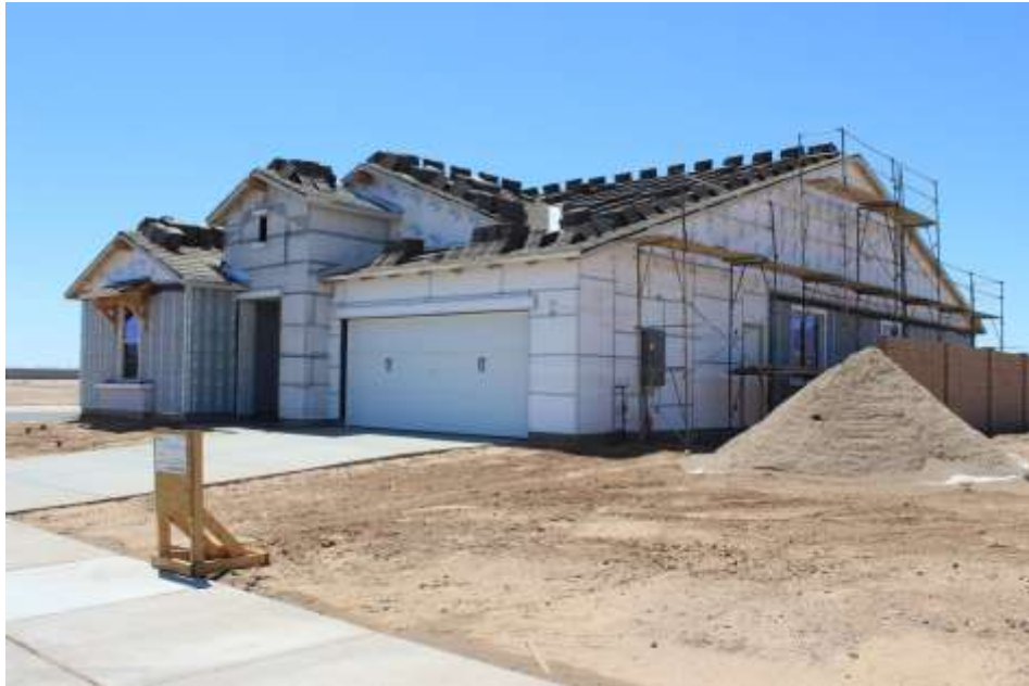
Figure 2: ICP walls assembled ready for finish
