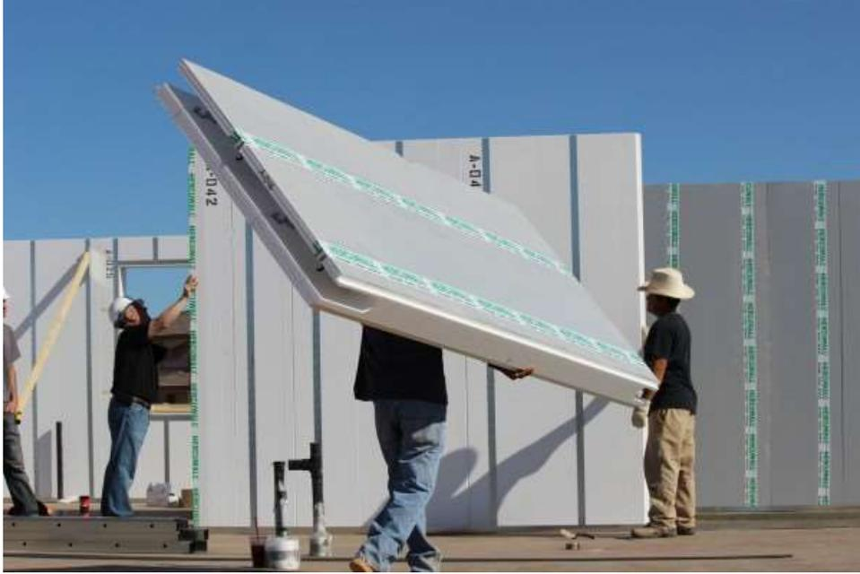
Figure 1: Lightweight panels easy to handle in the field
