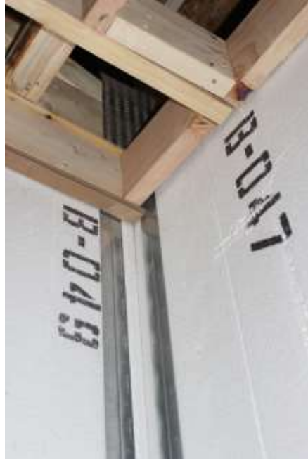
Figure 3: Numbered panels for easy assembly and raised heel construction
