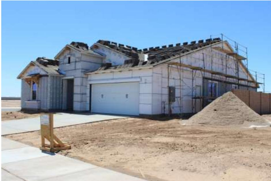
Figure 2: ICP walls assembled ready for finish
