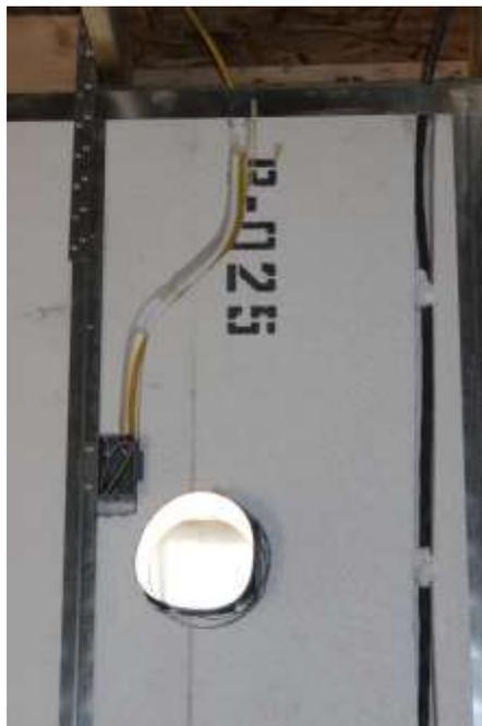
Figure 4: Electric wiring easily cut into foam panel
