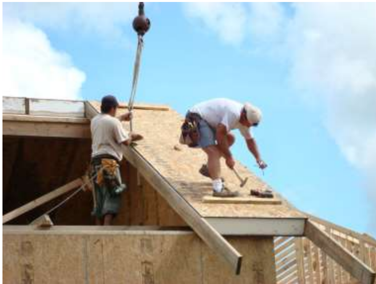
Figure 2: Carl Franklin Homes constructing roofs with crane set SIP panels.
