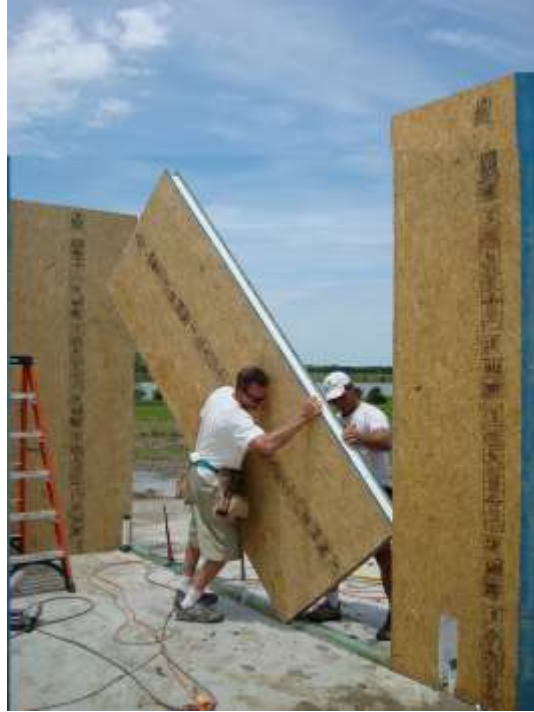
Figure 1: Carl Franklin Homes constructing walls with 4' SIP wall panels.
