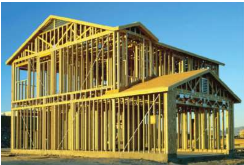
Figure 2: Typical wood frame structure from Architecture Curriculum at McGill University in Canada
